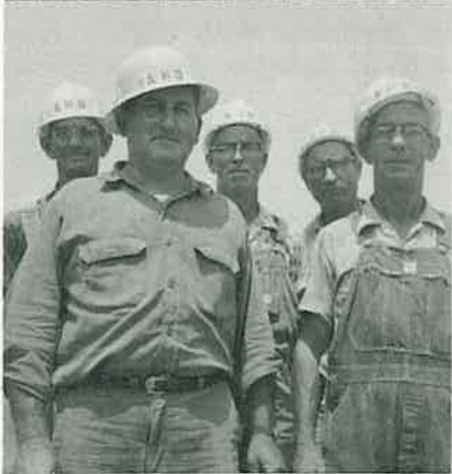
Part of the bridge crew in District 7 are (front): J. M. Renfro, S. B. Evans; (back), G. B. Glass, Clyde Coston, and John Core.
