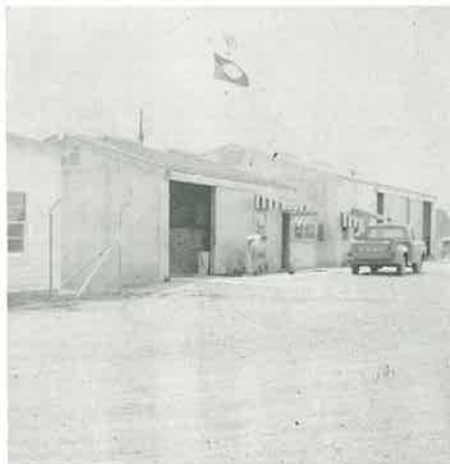
Above is the new resident engineer's office, job superintendent's office and maintenance area building at the Ouachita County area headquarters.
